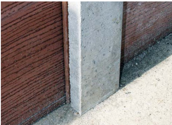
Concrete post cemented into position in the usual way
