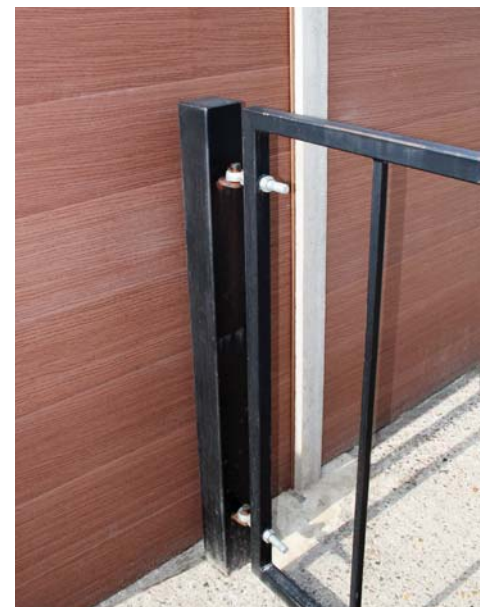
Typical steel gate posts can be cemented in separately
